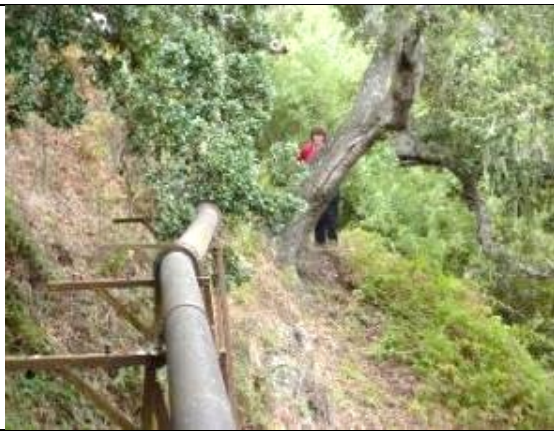
Photo: View gravity pipe in Carmel easement
