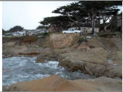
Photo: Looking at Pump Station Exterior
