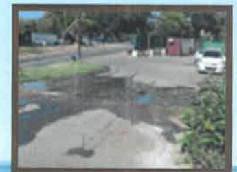
Leaking Sewer Main
