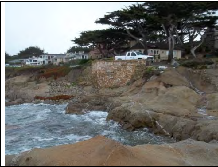
Photo: Looking at Pump Station Exterior
