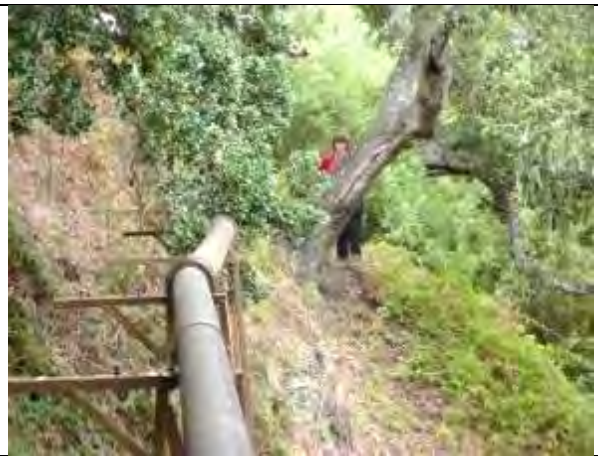
Photo: View gravity pipe in Carmel easement
