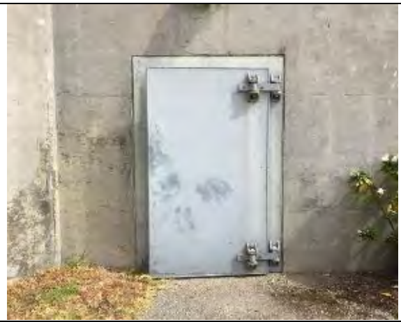
Photo: Old Flood Door in Headworks Basement
