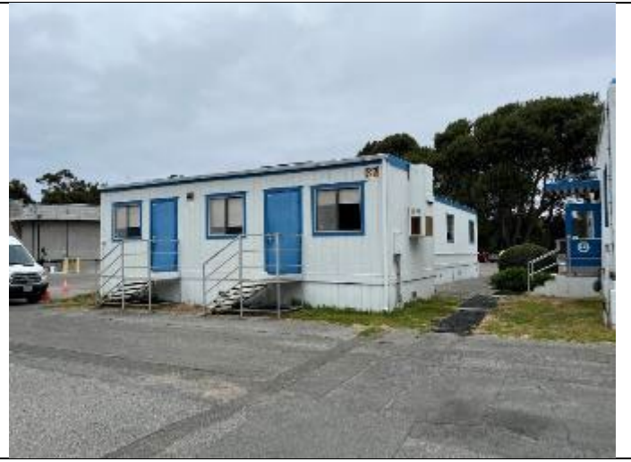
Photo: Office trailers at WWTP
