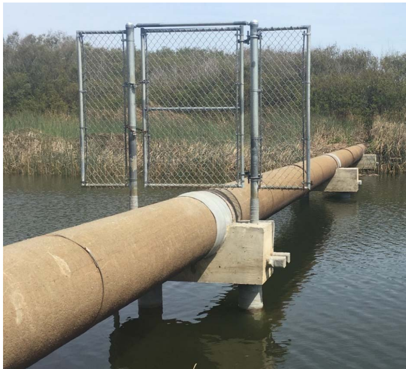
Photo of Completed Repair
