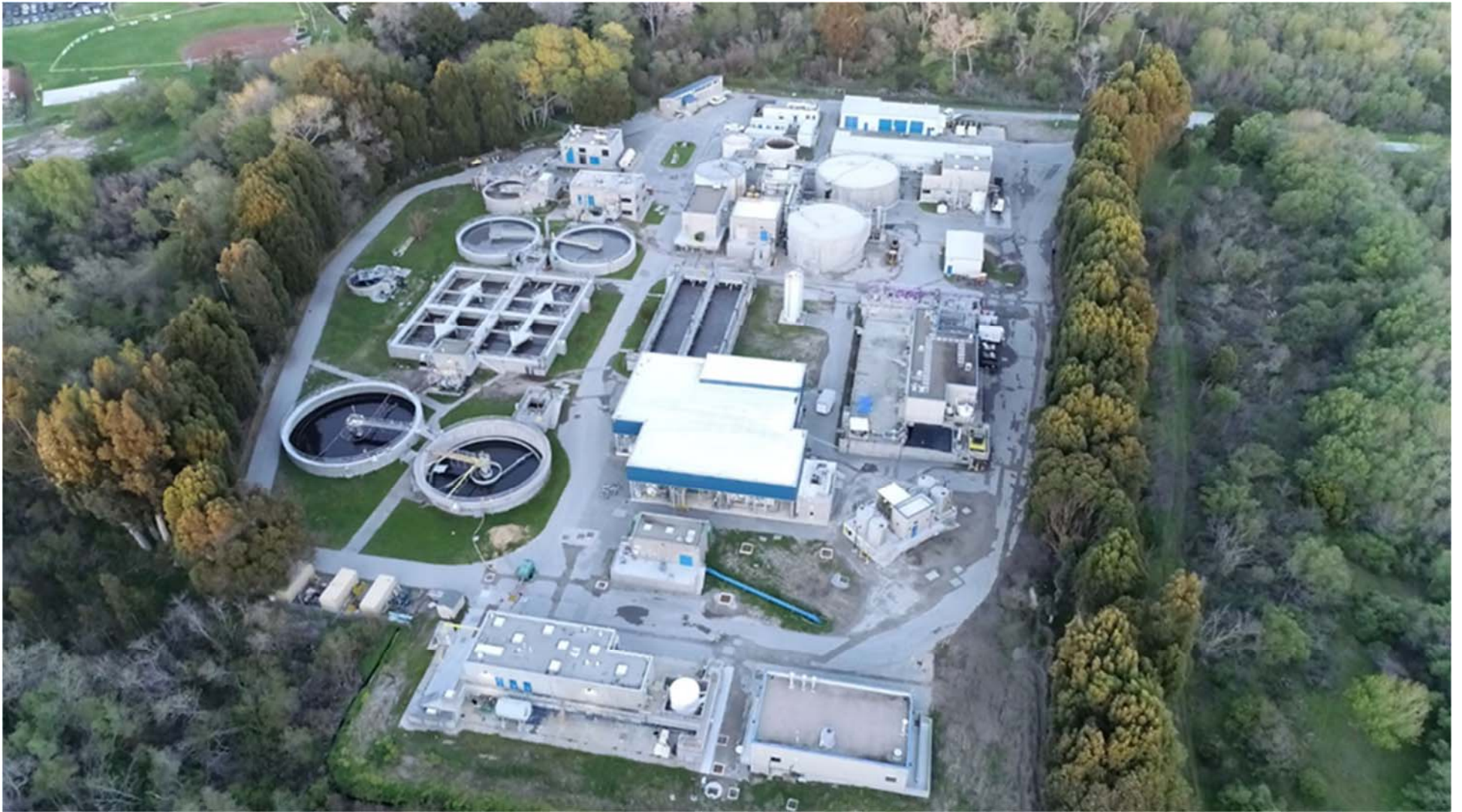
Figure 8 - CAWD WWTP Aerial
