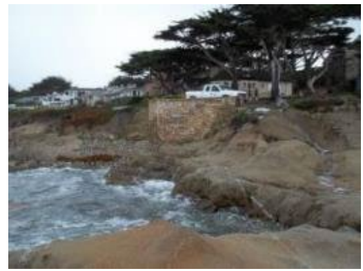
Photo: Looking at Pump Station Exterior
