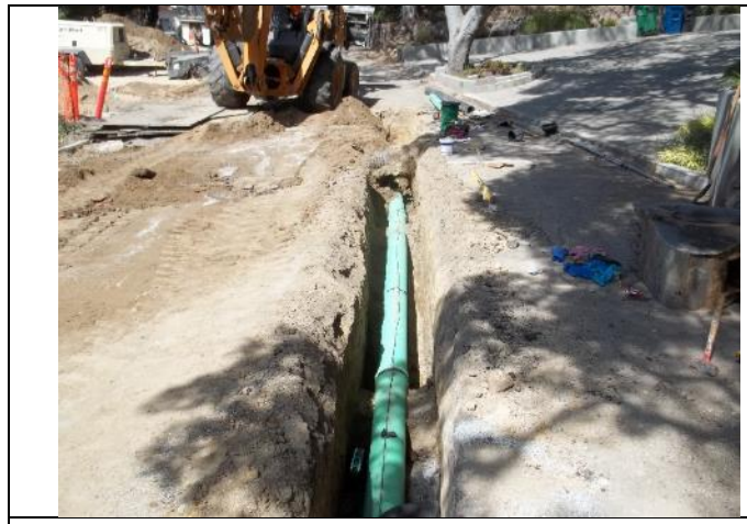
Photo: Sewer Line Repair
