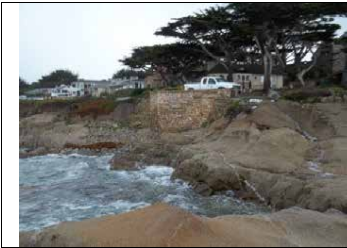
Photo: Looking at Pump Station Exterior
