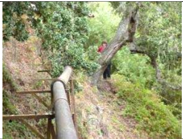
Photo: View gravity pipe in Carmel easement
