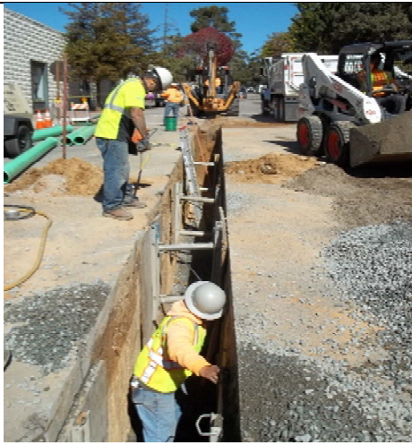
Photo: View of sewer line being replaced
