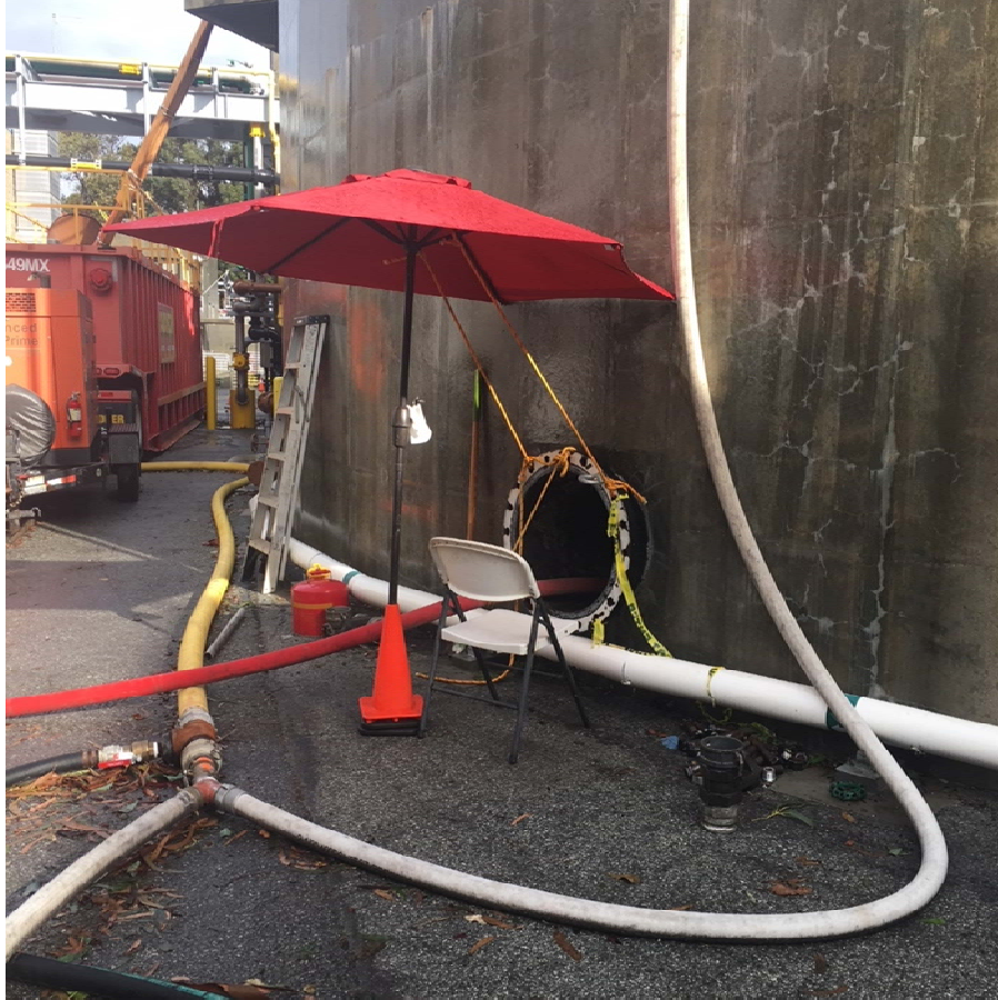
Photo 3: Side Hatch Access
