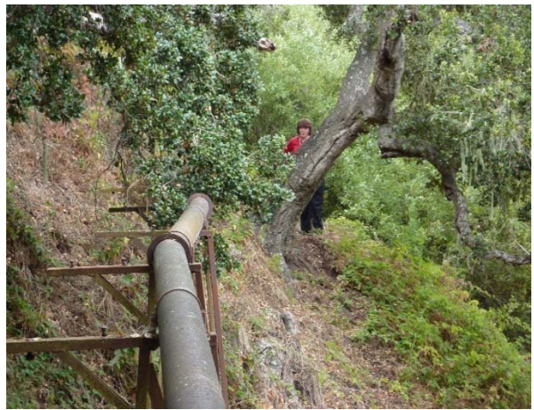
Photo: View gravity pipe in Carmel easement
