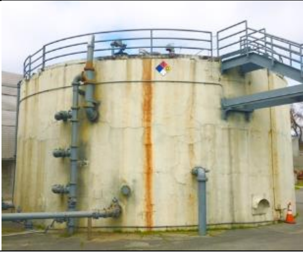
Photo: Old Digester No. 2
