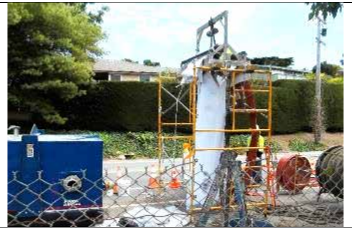
Photo: View CIPP Liner being installed
