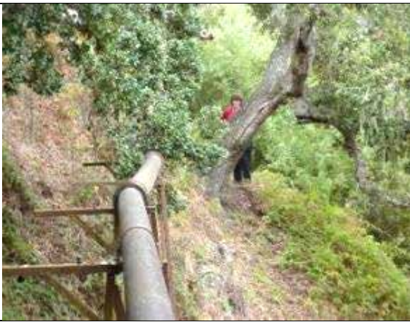
Photo: View gravity pipe in Carmel easement
