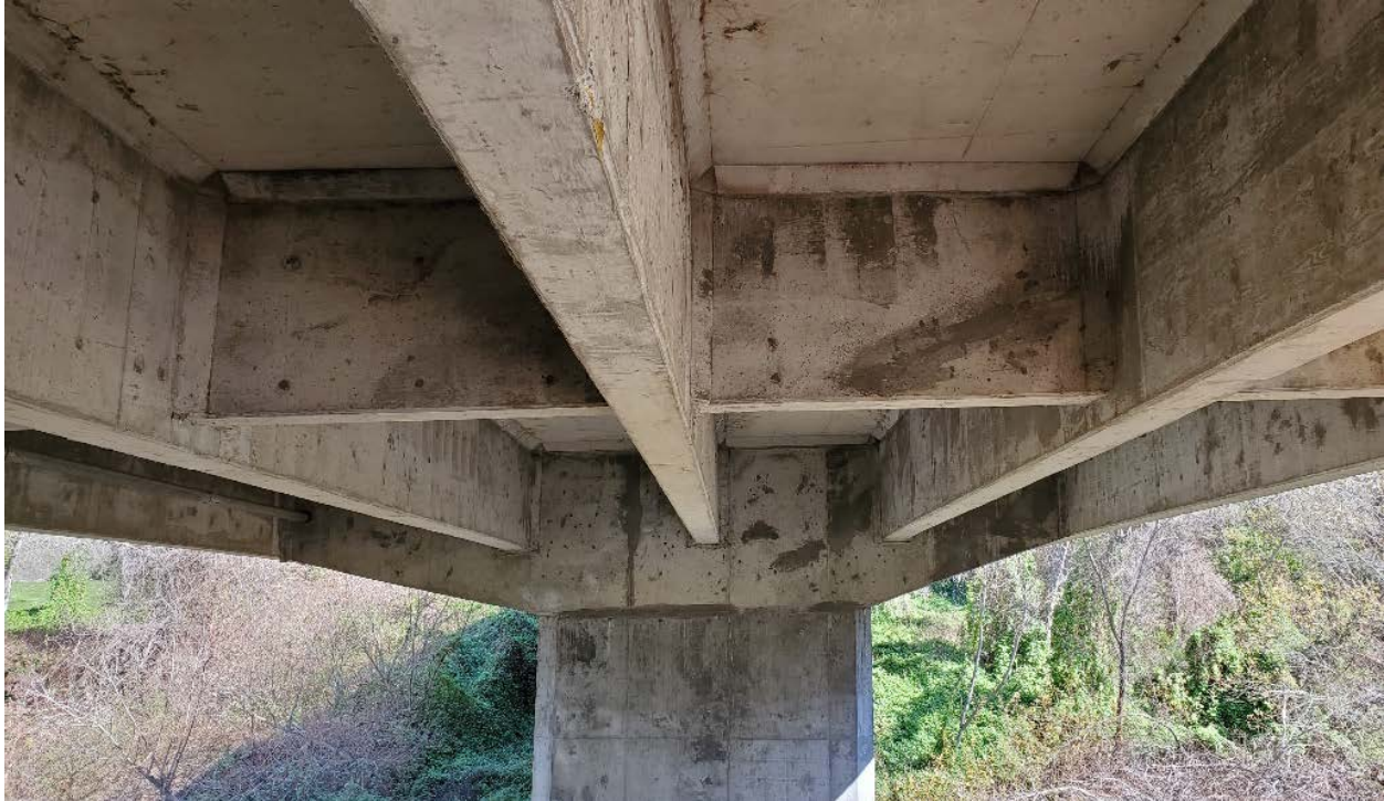
Photograph 3. The underside of the bridge at Valley Greens Drive, facing west.
