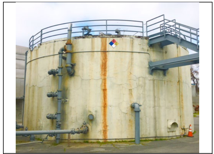
Photo: Old Digester No. 2
