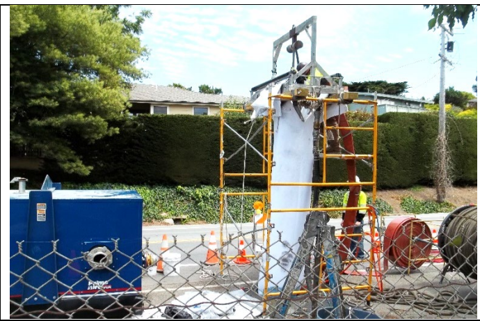
Photo: View CIPP Liner being installed
