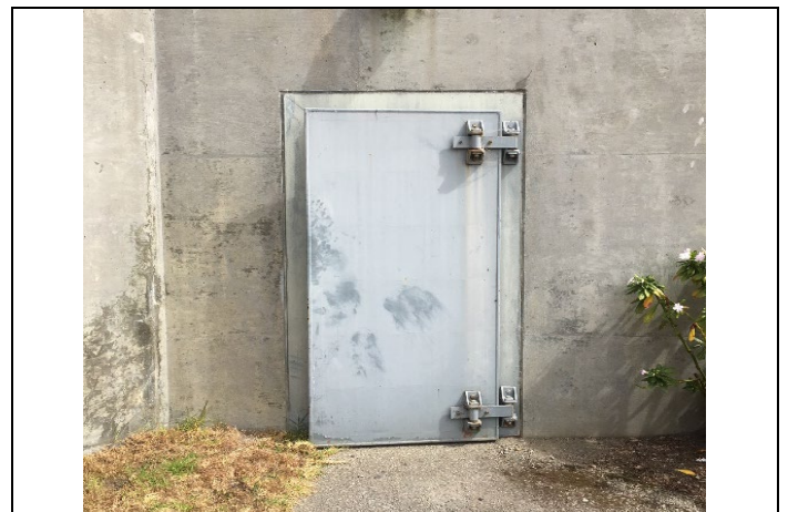
Photo: Old Flood Door in Headworks Basement
