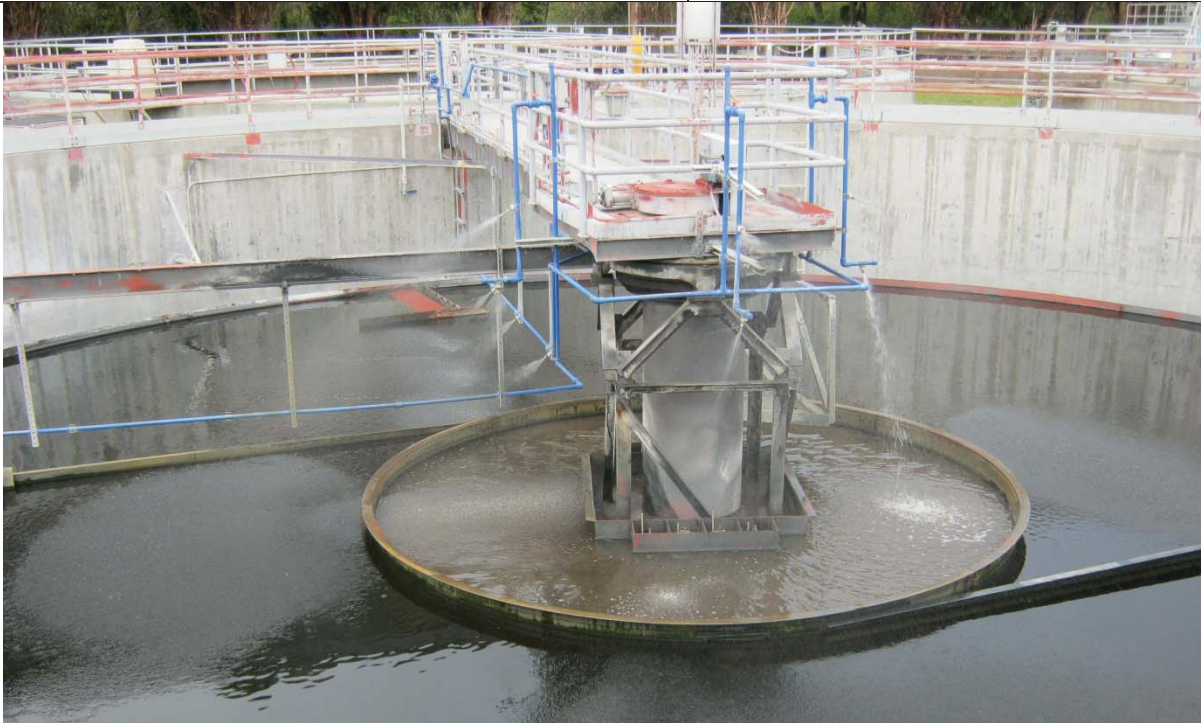
Secondary Clarifier Center Structure
