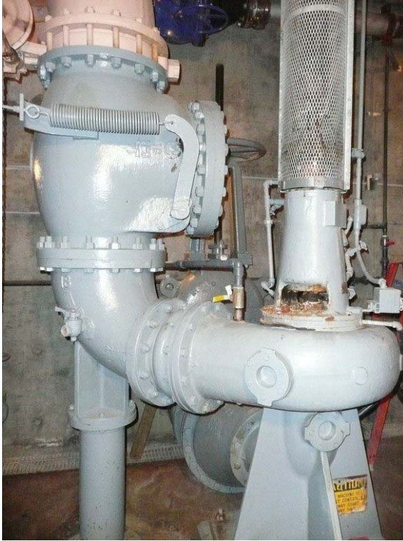
Figure 4: High-Service Pumps
