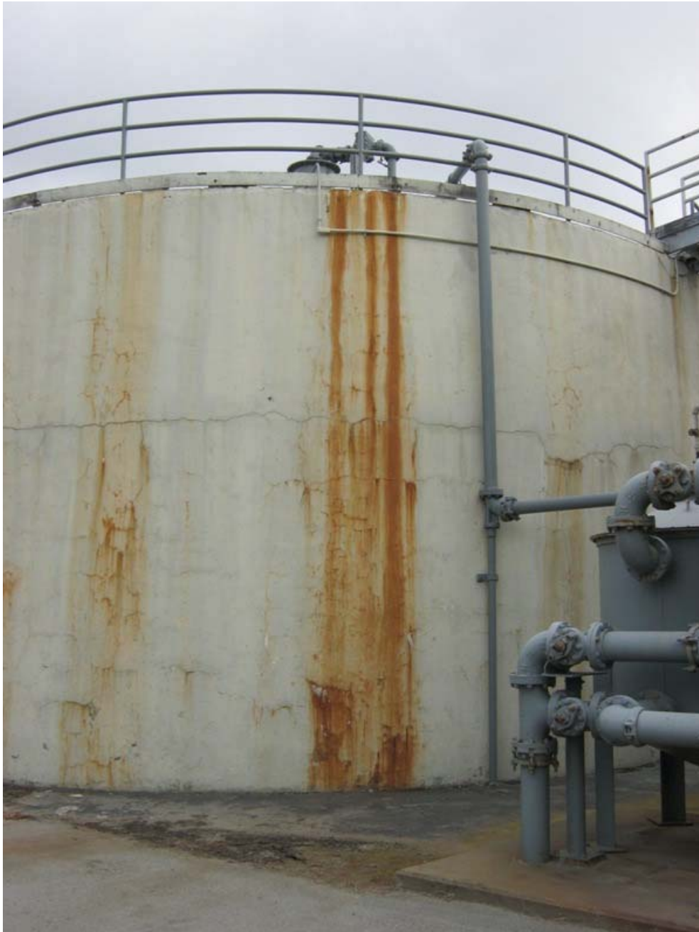
Figure 1: Digester 2 Exterior Wall
