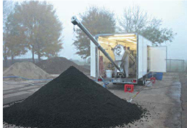
Contract dewatering with a trailer-mounted unit size 440
