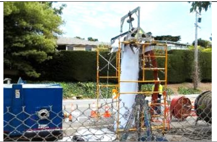
Photo: View CIPP Liner being installed
