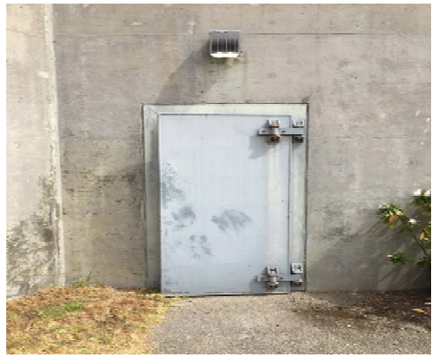
Photo: Old Flood Door in Headworks Basement
