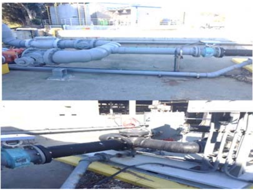
Photo: Existing Pipe (Left); New Pipe Example (Right)
