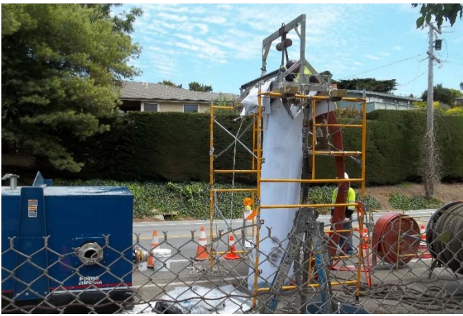
Photo: View CIPP Liner being installed
