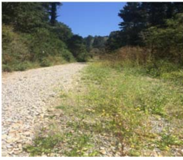
Photo: View of portion of Hatton Canyon Access Road that was repaired to allow access for construction equipment
