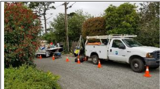
Photo: Pipe Repairs
