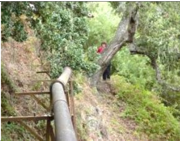
Photo: View gravity pipe in Carmel easement
