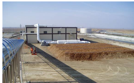
South Kern Compost Manufacturing Facility. Synagro utilizes an enclosed biosolids receiving and mixing building along with biofiltration in its compost system that controls VOCs and odors for the surrounding area.
