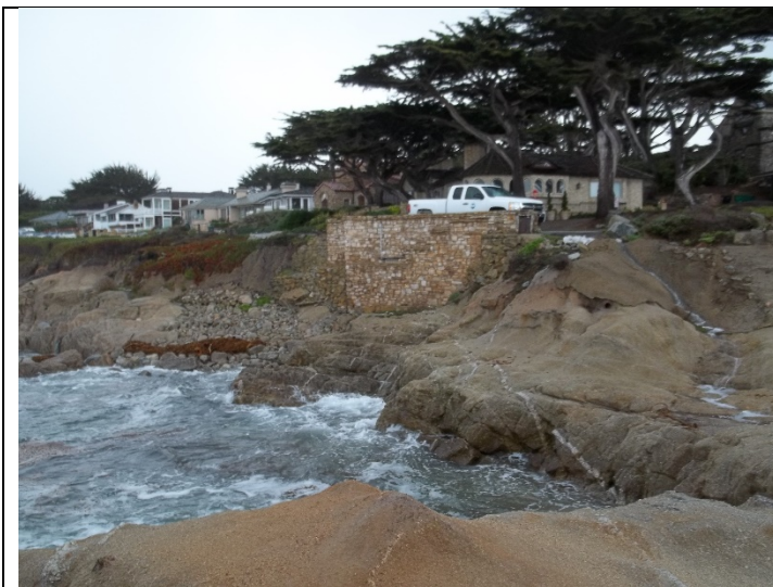
Photo: Looking at Pump Station Exterior
