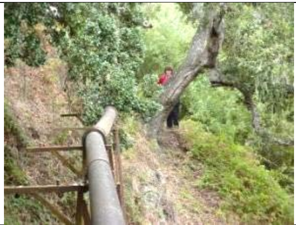
Photo: View gravity pipe in Carmel easement
