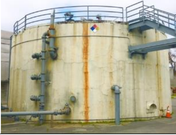
Photo: Old Digester No. 2
