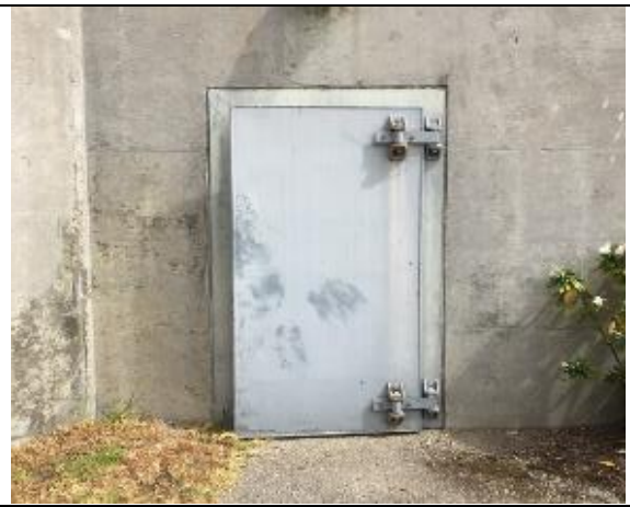
Photo: Old Flood Door in Headworks Basement
