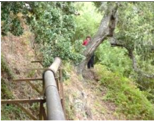
Photo: View gravity pipe in Carmel easement
