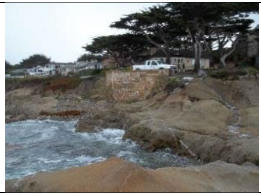
Photo: Looking at Pump Station Exterior
