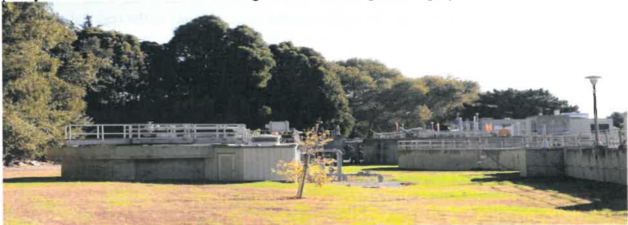
Clarifiers tanks & DAFT
