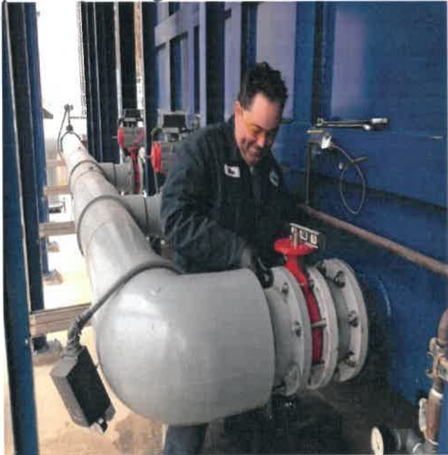
Repairs at Reclamation
