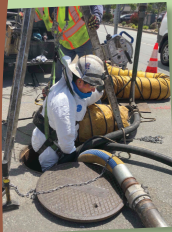
Rio Road construction caption
