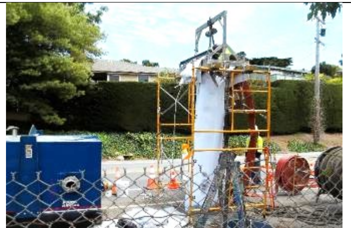
Photo: View CIPP Liner being installed
