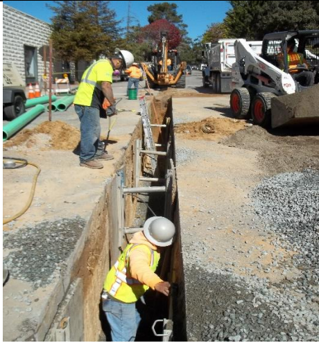
Photo: View of sewer line being replaced
