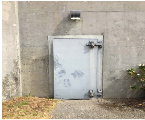
Photo: Old Flood Door in Headworks Basement
