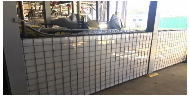
Photo: Sound Barriers partially installed around High Pressure RO Pumps
