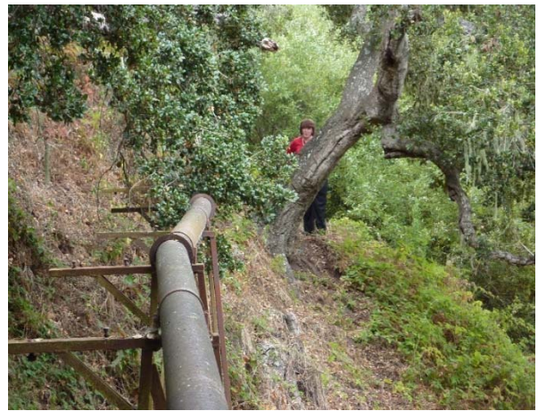
Photo: View gravity pipe in Carmel easement
