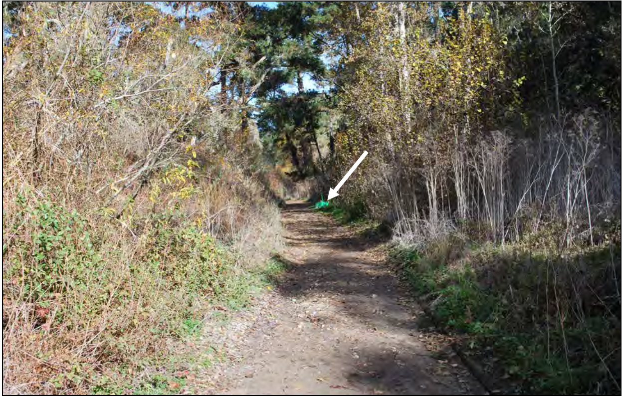
Figure 8: Hatton Canyon Trail with sewer manhole P805 – view north
