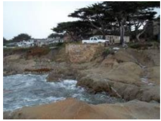
Photo: Looking at Pump Station Exterior
