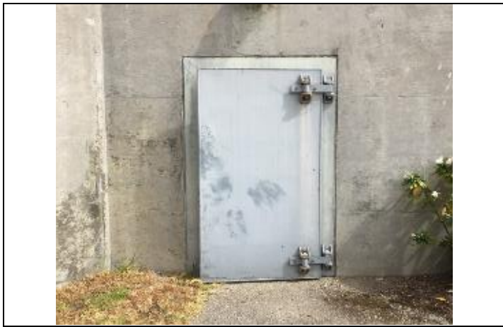
Photo: Old Flood Door in Headworks Basement
