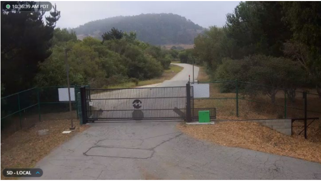
Photo: Security Cameras – Plant Gate View
