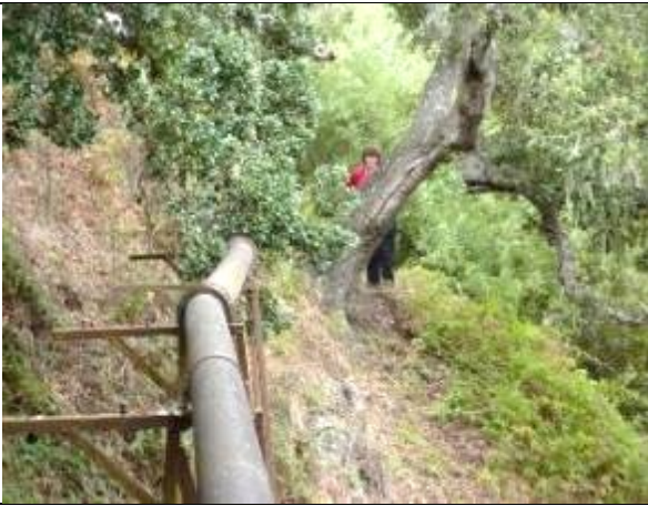
Photo: View gravity pipe in Carmel easement
