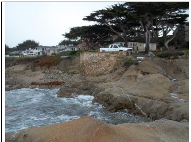
Photo: Looking at Pump Station Exterior
