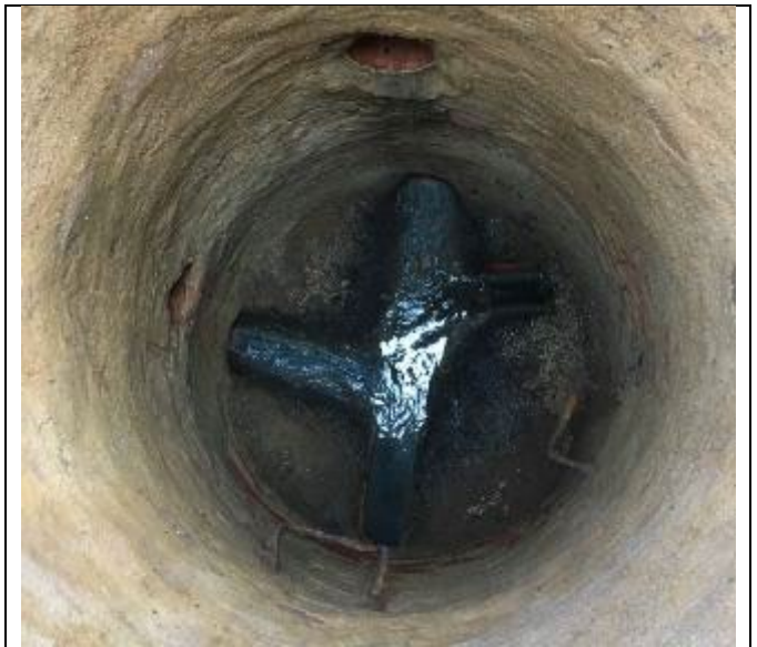
Photo: Inside of Sewer Manhole
