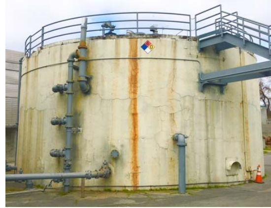
Photo: Old Digester No. 2
