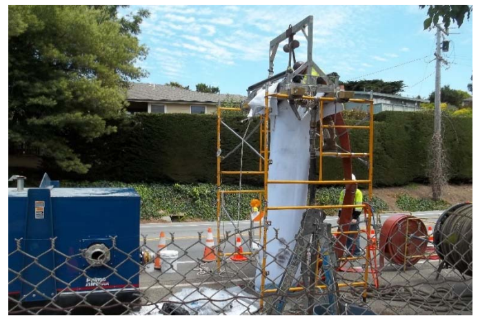
Photo: View CIPP Liner being installed
