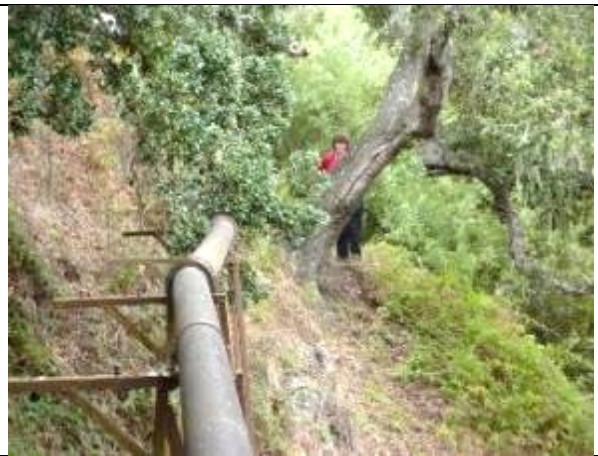
Photo: View gravity pipe in Carmel easement
