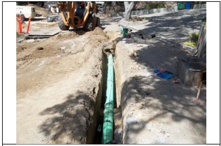
Photo: Sewer Line Repair
