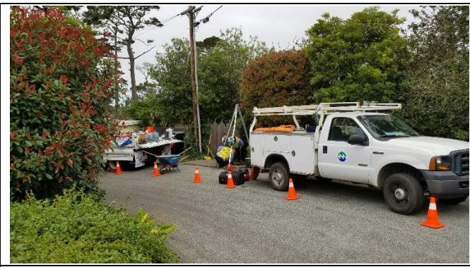
Photo: Pipe Repairs
