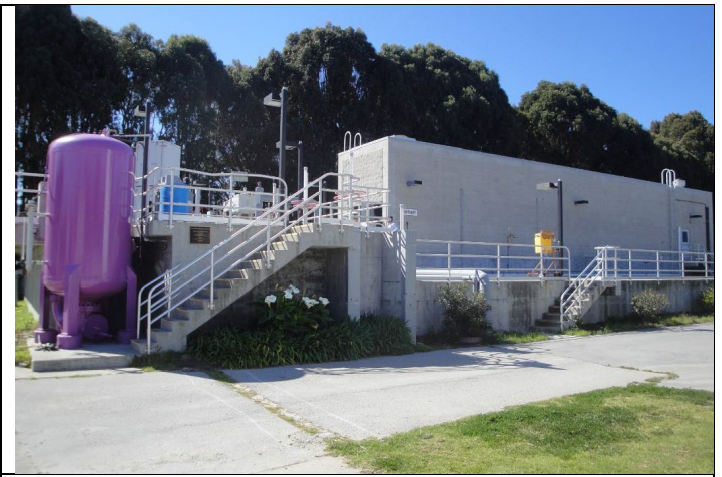
Photo: Exterior of Tertiary Building
