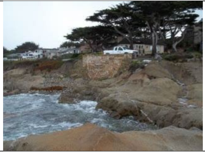
Photo: Looking at Pump Station Exterior
