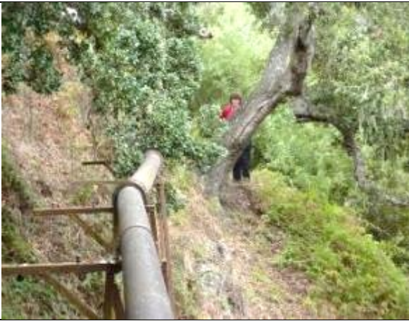
Photo: View gravity pipe in Carmel easement
