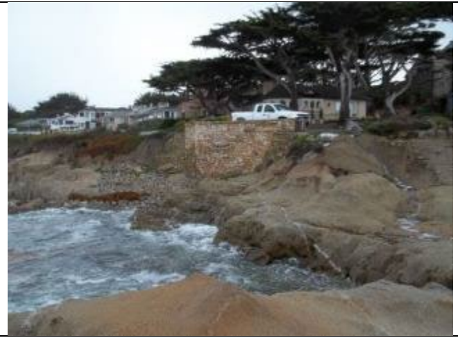
Photo: Looking at Pump Station Exterior
