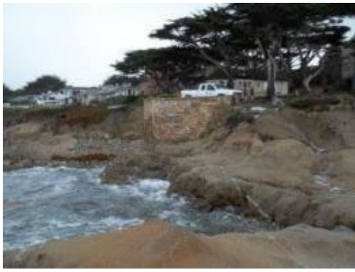
Photo: Looking at Pump Station Exterior
