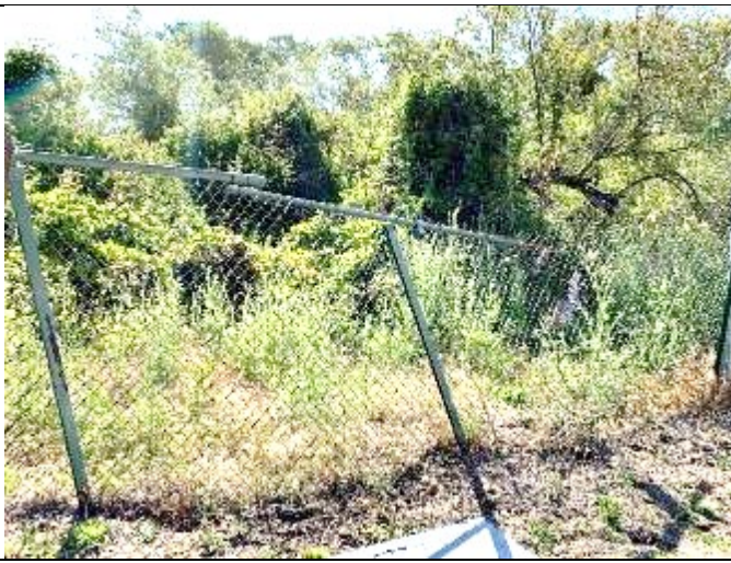
Photo: Existing dilapidated fence
