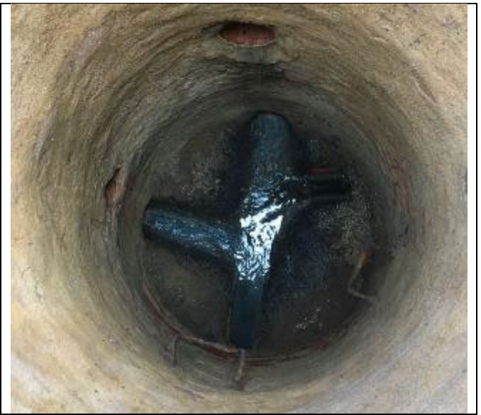
Photo: Inside of Sewer Manhole
