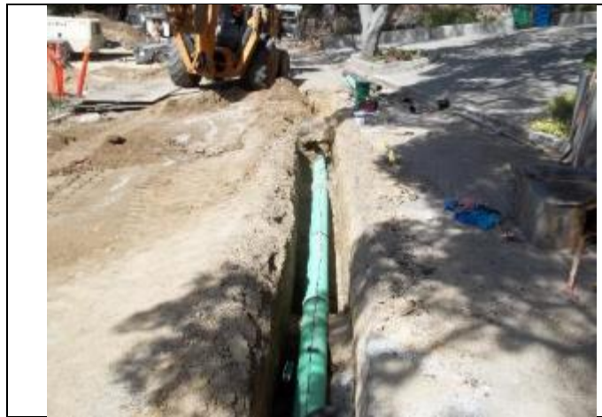
Photo: Sewer Line Repair
