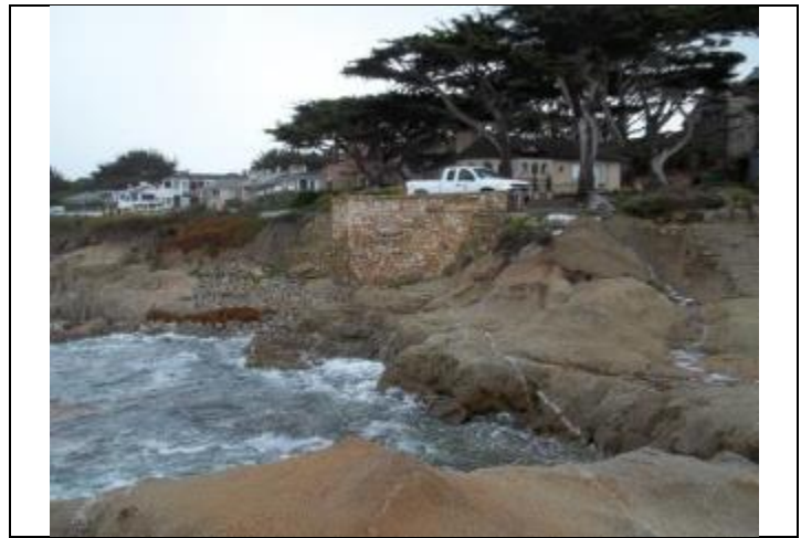
Photo: Looking at Pump Station Exterior
