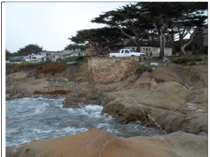
Photo: Looking at Pump Station Exterior
