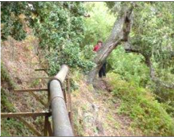
Photo: View gravity pipe in Carmel easement
