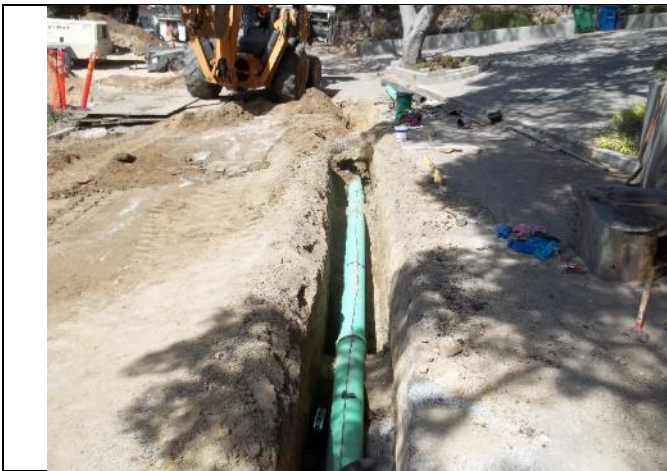
Photo: Sewer Line Repair
