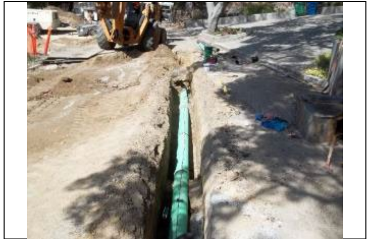
Photo: Sewer Line Repair
