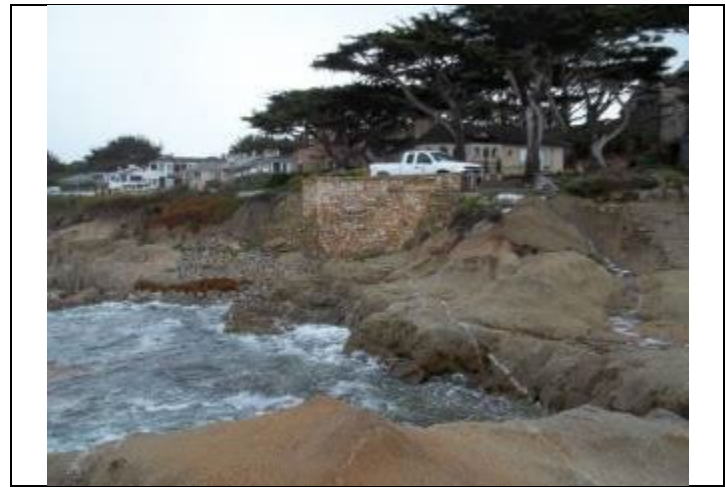
Photo: Looking at Pump Station Exterior
