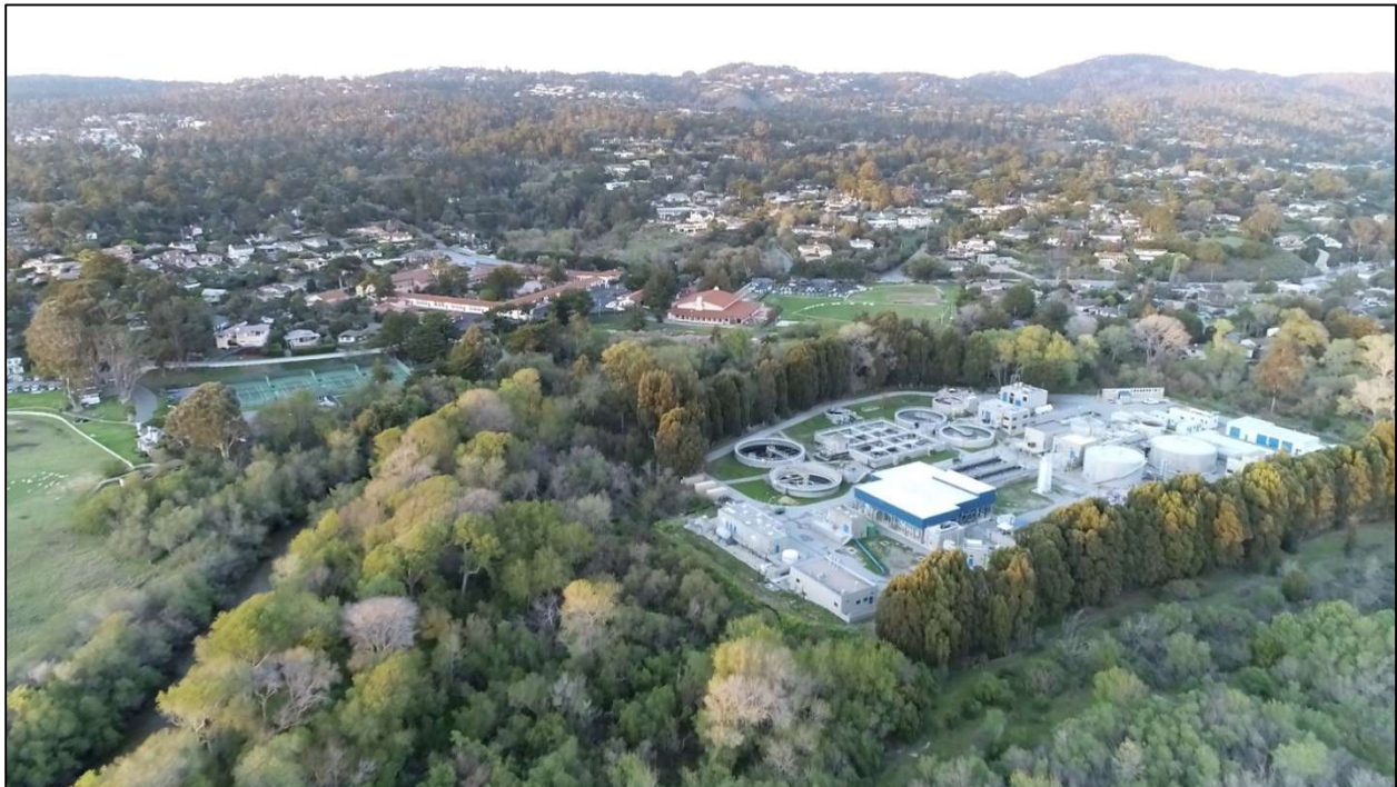
Figure: Aerial View of Carmel Area Wastewater District Wastewater Treatment Plant
