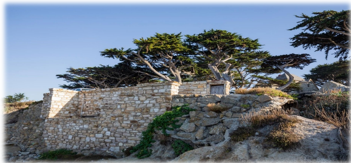
Bay & Scenic Pump Station
