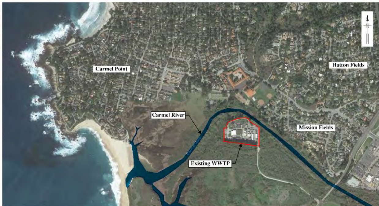
Figure 2-2: Aerial View of Existing CAWD WWTP and Surrounding Area
