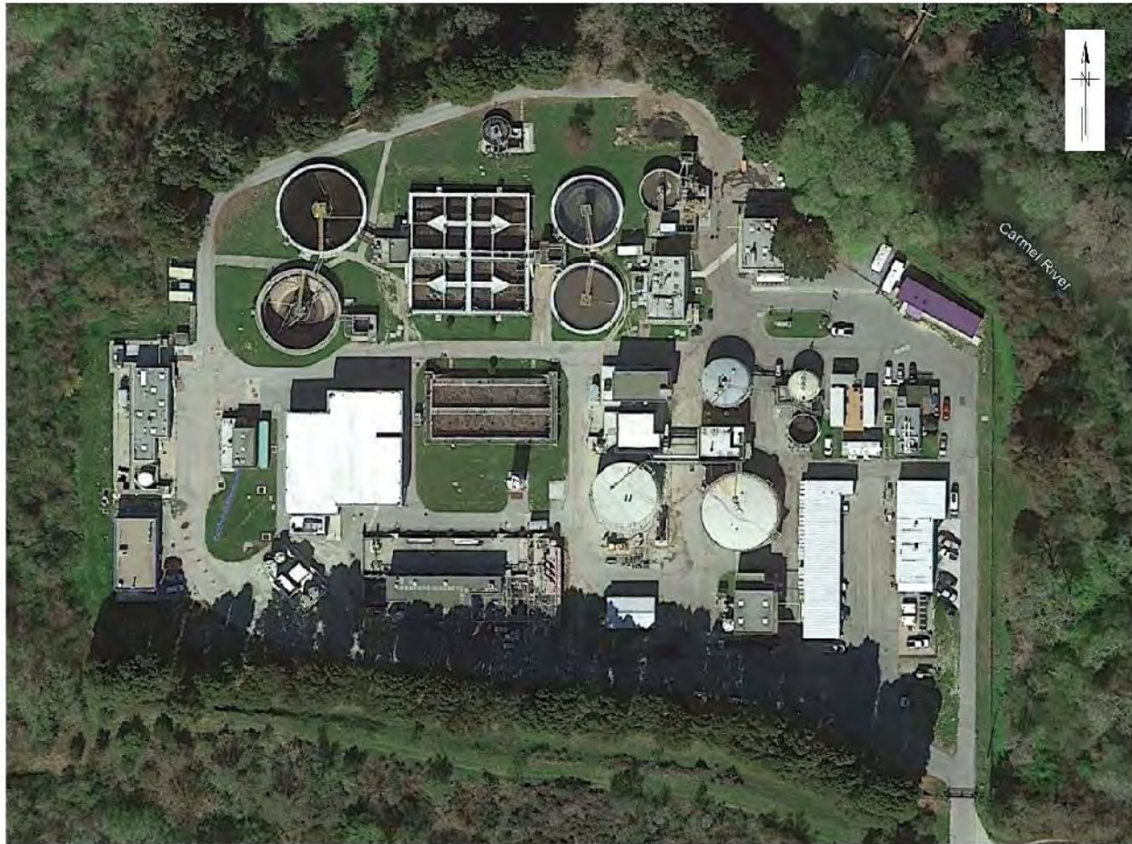
Figure 3-4: Existing CAWD WWTP
