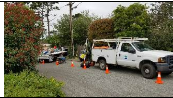
Photo: Pipe Repairs
