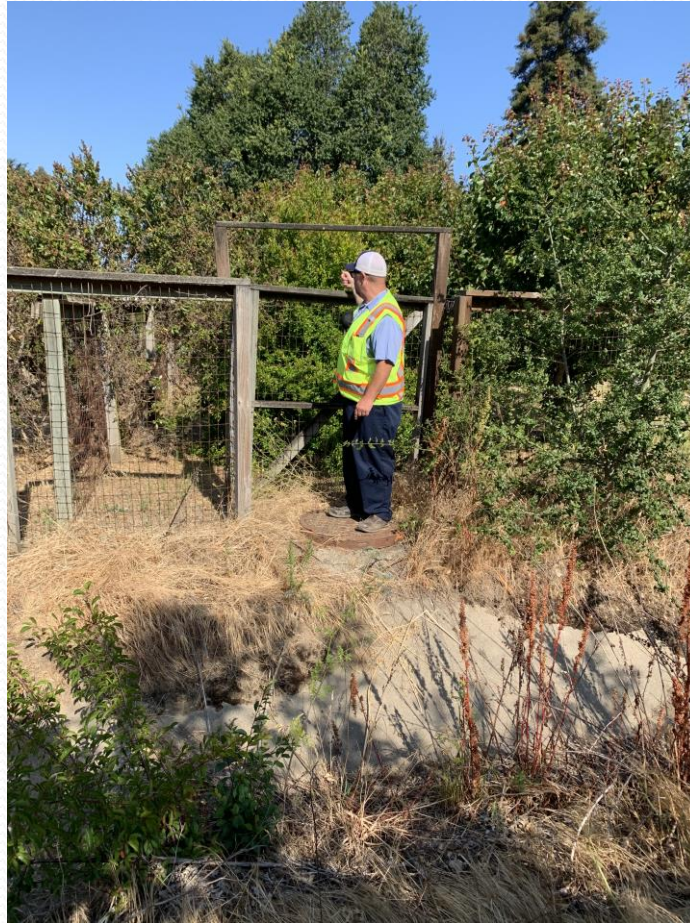
3 rd Manhole West of Via Petra
