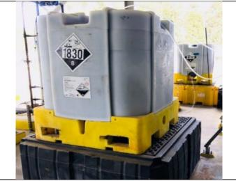
Photo: Existing totes used for Sulfuric Acid storage and Feed
