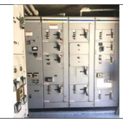
Photo: Existing Headworks Motor Control Center to Be Replaced in Project
