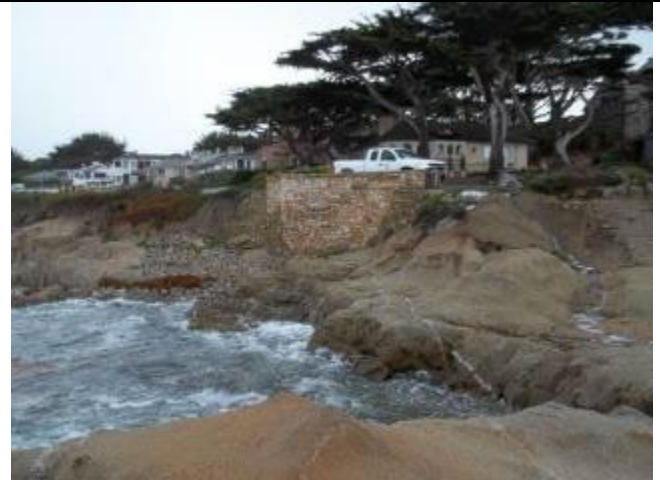
Photo: Looking at Pump Station Exterior
