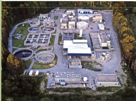
Aerial photo taken this April shows the CAWD treatment plant after construction of Phase One. Our community can rest assured knowing that our sophisticated treatment process produces one of the cleanest effluents in the state.
