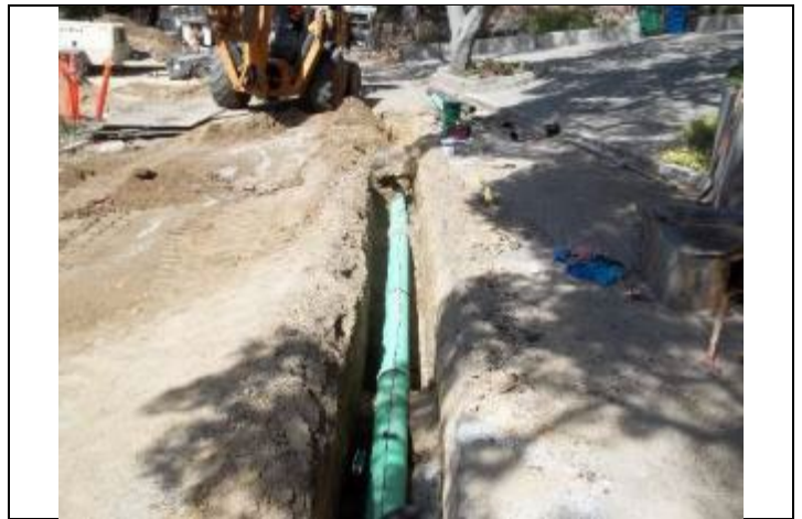
Photo: Sewer Line Repair
