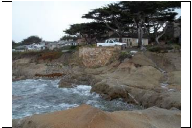
Photo: Looking at Pump Station Exterior
