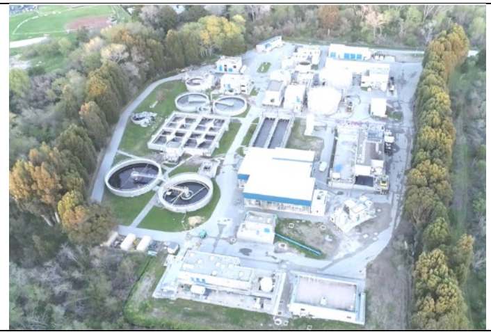
Photo: WWTP Aerial Showing Eucalyptus Trees Around Perimeter
