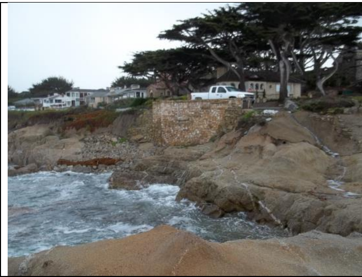
Photo: Looking at Pump Station Exterior
