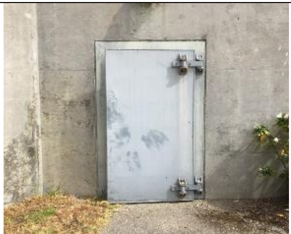
Photo: Old Flood Door in Headworks Basement
