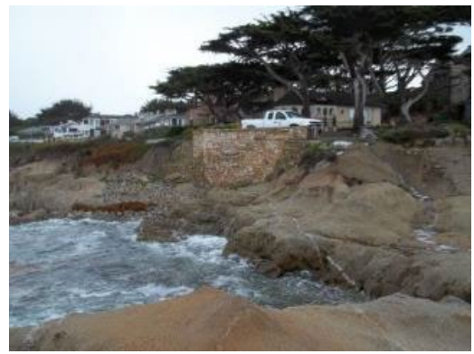
Photo: Looking at Pump Station Exterior
