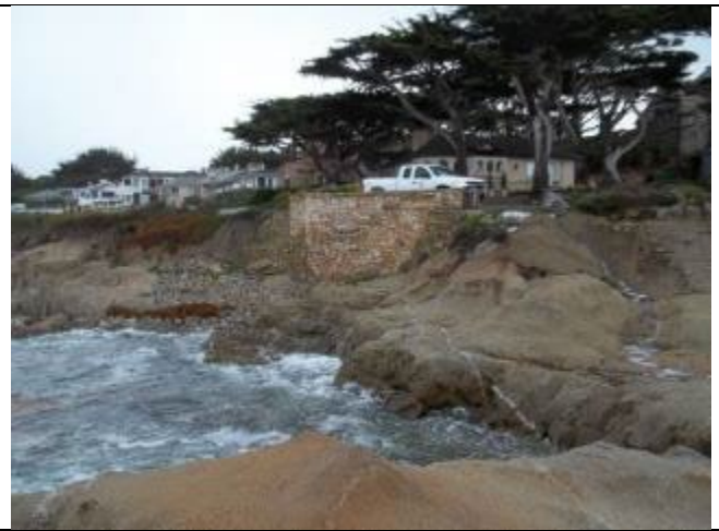
Photo: Looking at Pump Station Exterior
