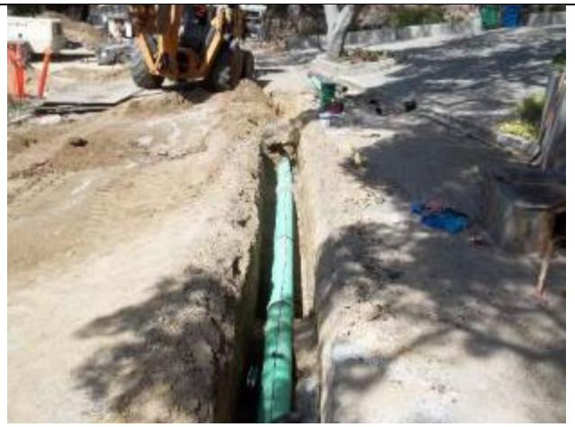
Photo: Sewer Line Repair
