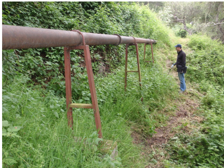
Photo 2 Reach 1 Facing northwest
