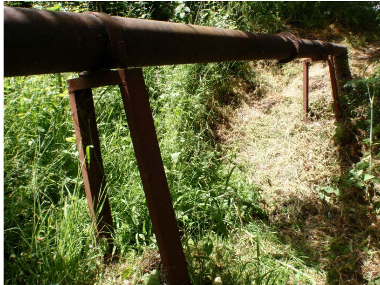
Photo 5 Reach 3 Elevated sewer line on C-channel supports
