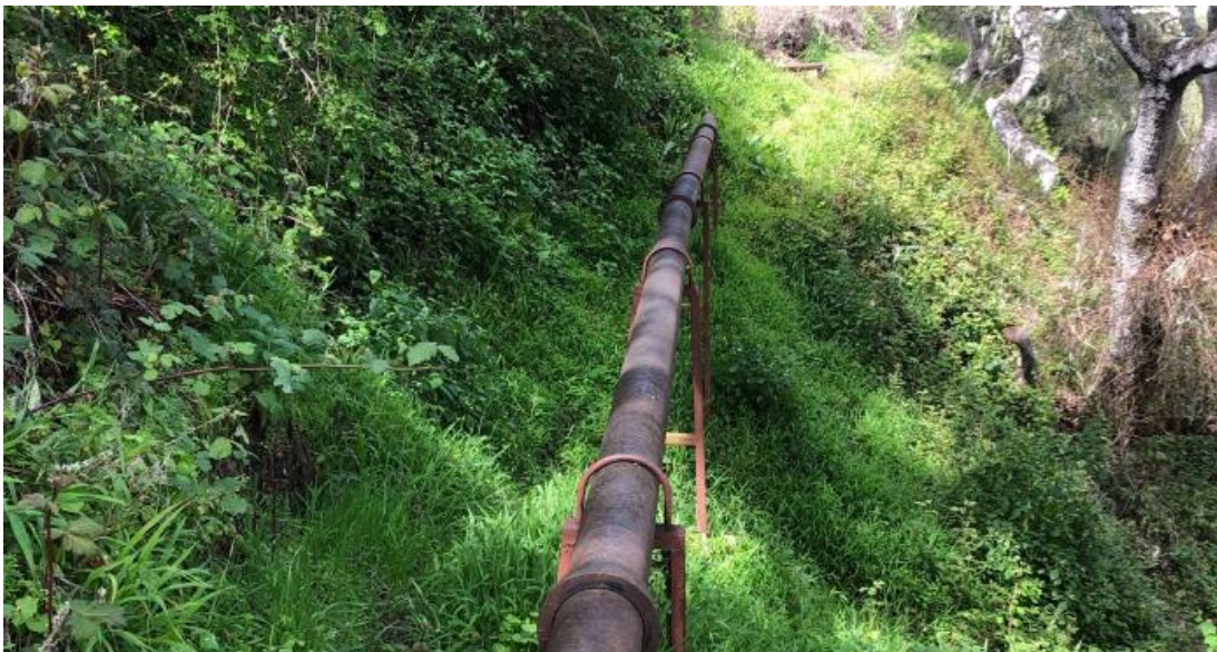
Figure 1. Aerial Portion of the Existing Interceptor
