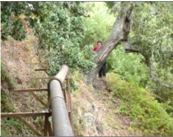
Photo: View gravity pipe in Carmel easement
